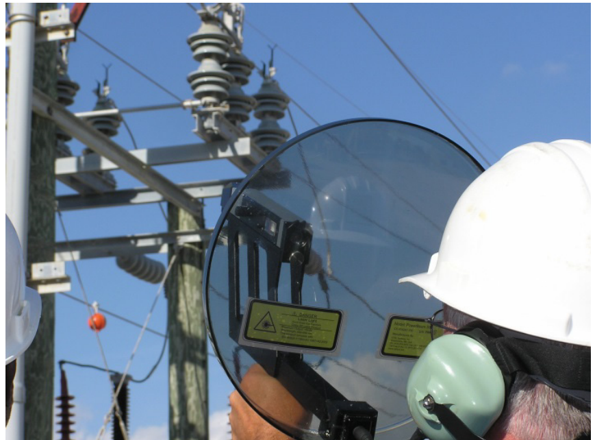
Figure 3. Ultrasound Detector with Parabolic Attachment for Detection of Corona Discharge
