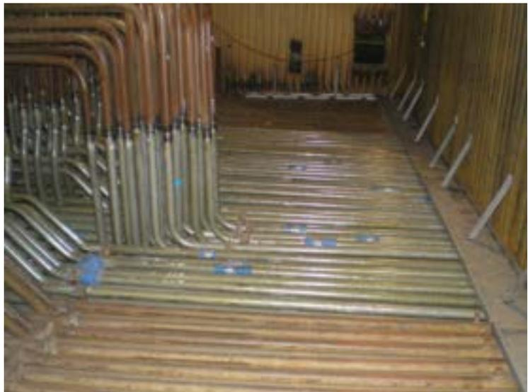
**Figure 1.** Inside view of the re-heater. The tube bundles are stacked more than 20 feet below.
