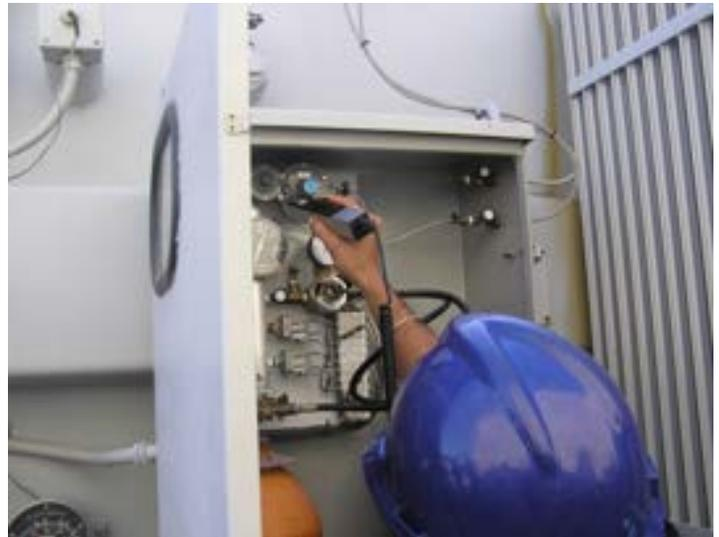
**Figure 3.** Ultrasound Detector being used to locate leak in transformer at substation
